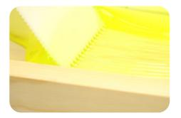
Measure and mix the resin and hardener before pouring out the mixture in one go and if required using a spreader to ensure full coverage.
