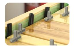
covered leave the resin to partially cure. Ideally you want to remove the tile spacers when the resin has started to gel whilst it is still easy to remove them. It can then be left to reach the B-stage again before moving on to stage 3 - the fill layer.
